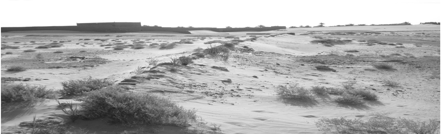
Figure 3. Seguia (canal) de la foggara Outakou (Timimoun) couverte de roches plates (REMINI, 2008). Seguia (channel) of the Outakou (Timimoun) foggara covered with flat rocks (REMINI, 2008).
